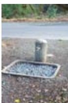
Water drains cleaned
