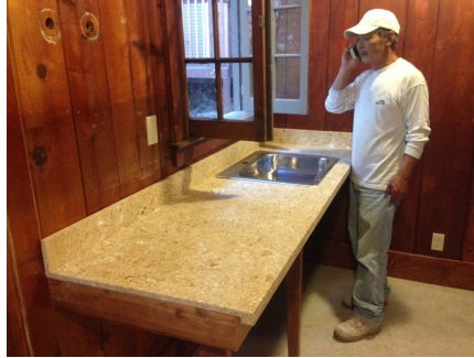
New countertop in Cabin 4 kitchen.
